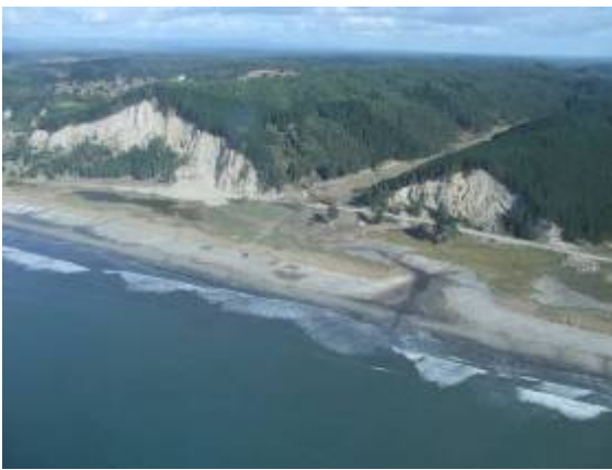
Photo 11 Slope failure at Las Peñas near Arauco
