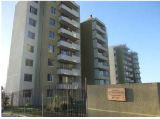
Photo 1 Tilting of apartment building at Los Presidentes
