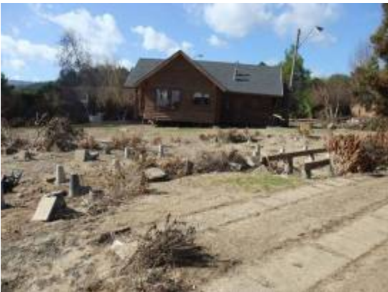
Photo 25 House that floated when tsunami came
