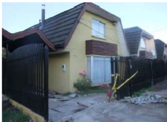
Photo 2 17-cm Subsidence of houses in Bayona, San Pedro de la Paz
