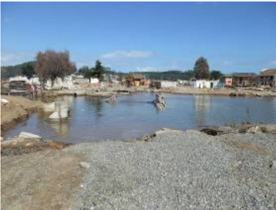
Photo 23 Tsunami-induced erosion in Dichato
