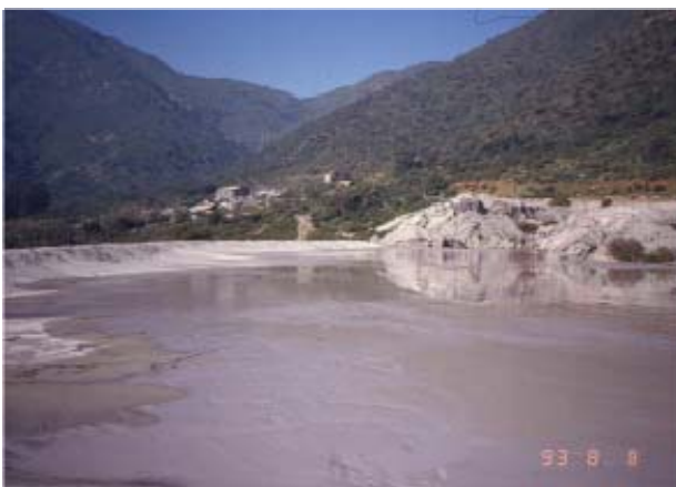
Photo 5 Reservoir of tailing dam at Veta del Agua in 1993.
