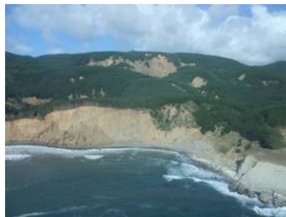
Photo 12 Slope failure at Lavapié
