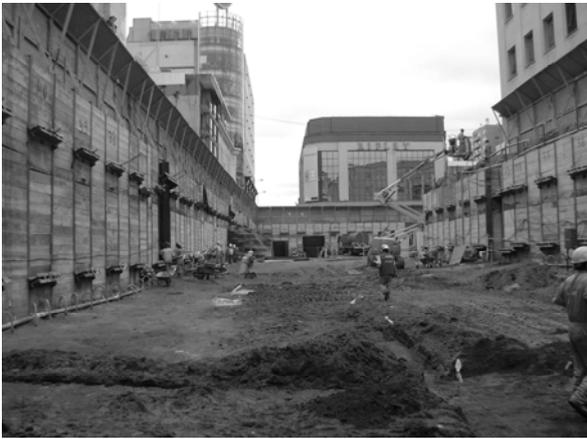
Figure 12: View of the excavation for the underground parking, showing SPW and well points
