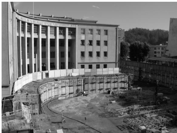
Figure 4: View of the curved anchored SPW adjacent to the Tribunals
