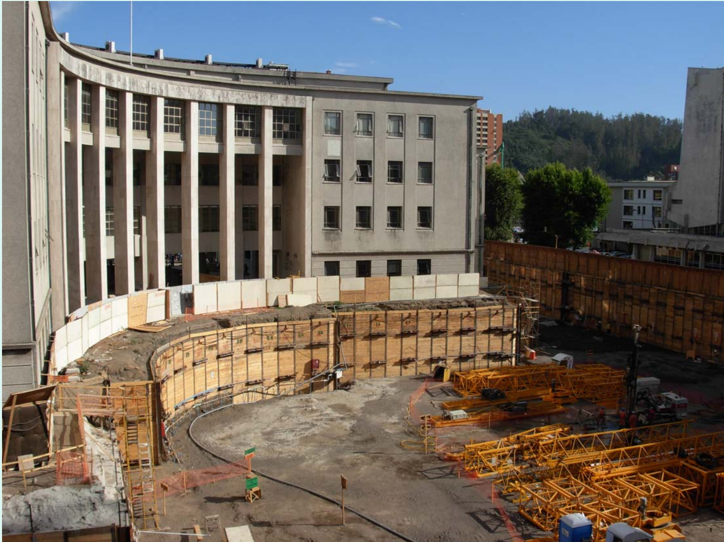
Curved anchored Soldier Pile Wall
