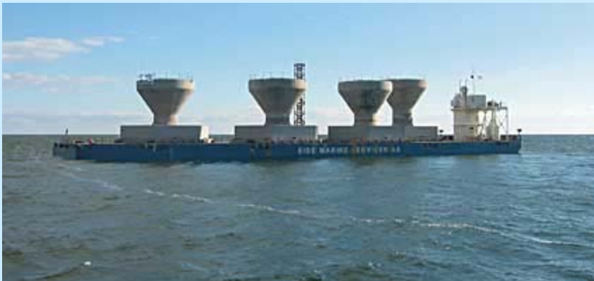
Gravity base foundations at Nysted
