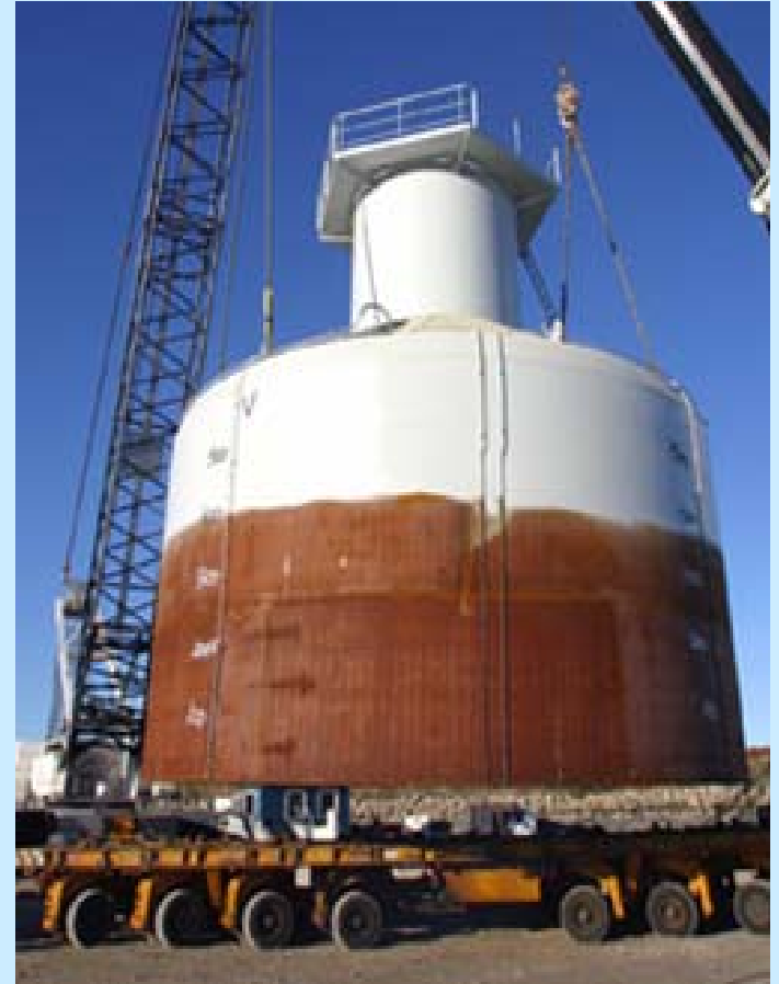
12 m diameter suction caisson
