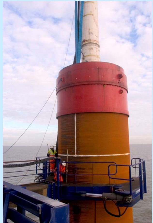
Monopile foundation at Kentish Flats
