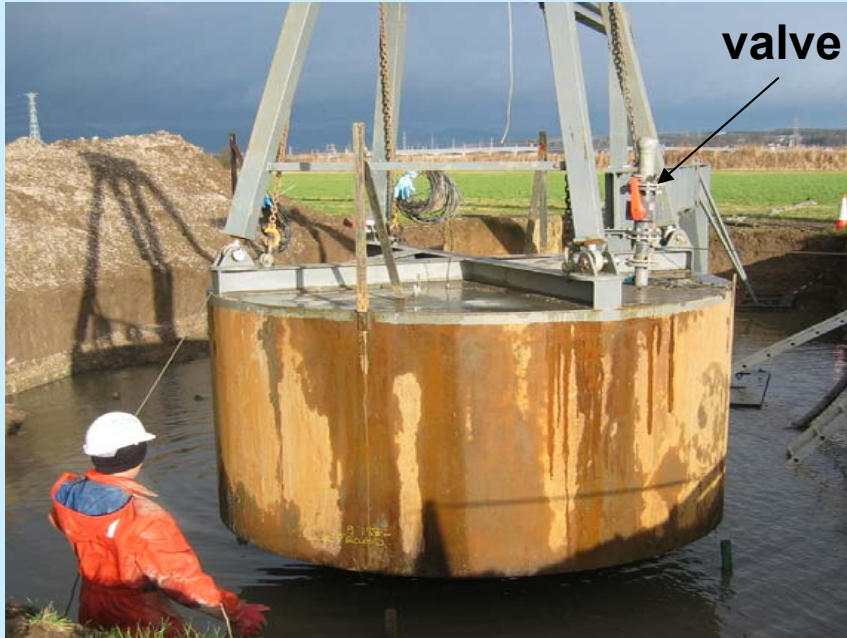
3 m diameter suction caisson
