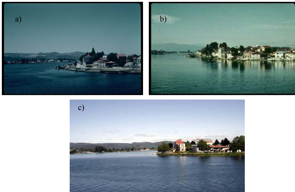
Figure 6: View of Valdivia from the Teja Island (a) before the 1960 earthquake, (b) immediately after (Steinbrugge and Flores, 1963) and (c) nowadays
