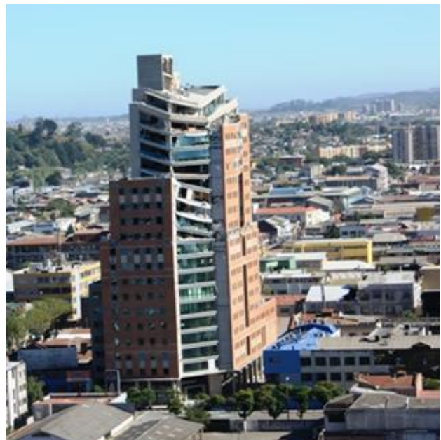
Figure 5. O’Higgins Tower, collapsed from tenth floor upwards, at Concepción.
