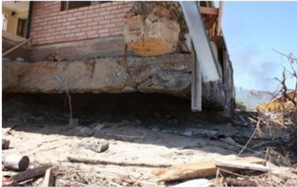
Figure 19. Intact foundation and superstructure of a house that was submitted to the tsunami in Dichato.
