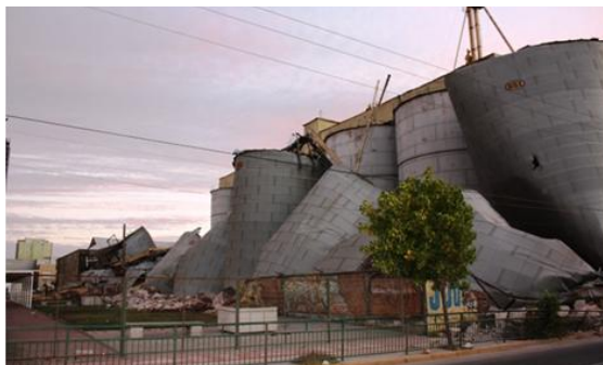
Figure 2. Silos that failed at center of Concepción.
