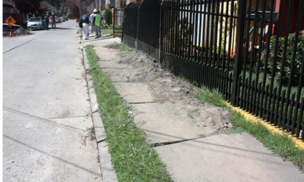
Figure 11. Generalized liquefaction in a group of single family homes. San Pedro La Paz.
