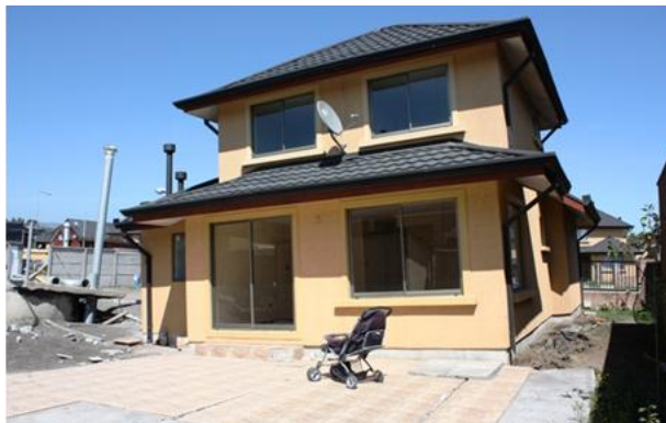
Figure 12. Heavy sinking and collapse in a single family home due to liquefaction.
