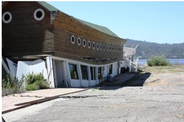
Figure 16. Extended cracking on the bank of the Bío Bío river.
