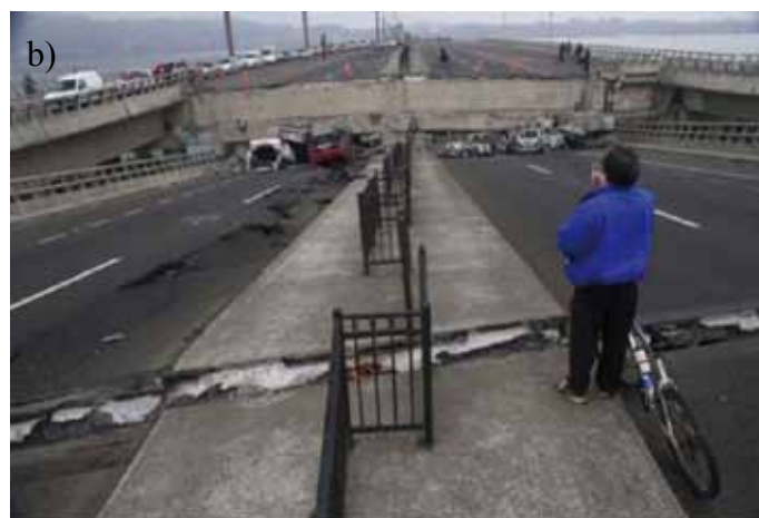
Figure 10: a) Abutment settlement and lateral displacement in Concepción railway bridge and b) collapse in the access to the Llacolén bridge in the Concepción side
