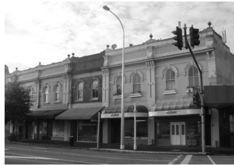
Figure 2: Jervois Road, Auckland, New Zealand.
