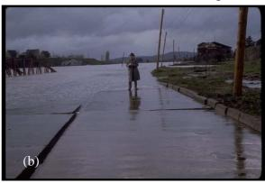
Figure 3: Road along the promenade showing concrete pavement distorted, broken and tilted towards the river (a) under Pedro de Valdivia Bridge and (b) passing the bridge upstream (Steinbrugge and Flores, 1963)
